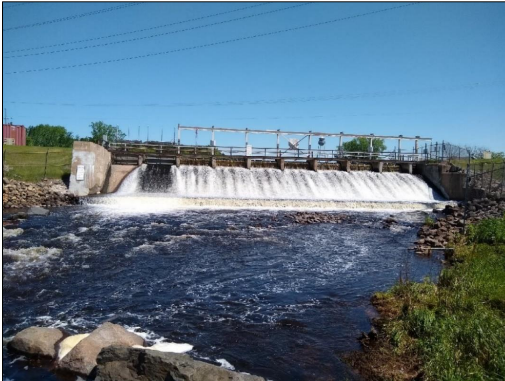
Figure 4.10.1-1 View of the Hayward Dam Spillway looking upstream from bypass reach.
