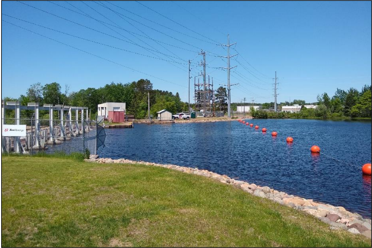
Figure 4.10.1-2 Hayward Dam and powerhouse from the East Bank (looking west)
